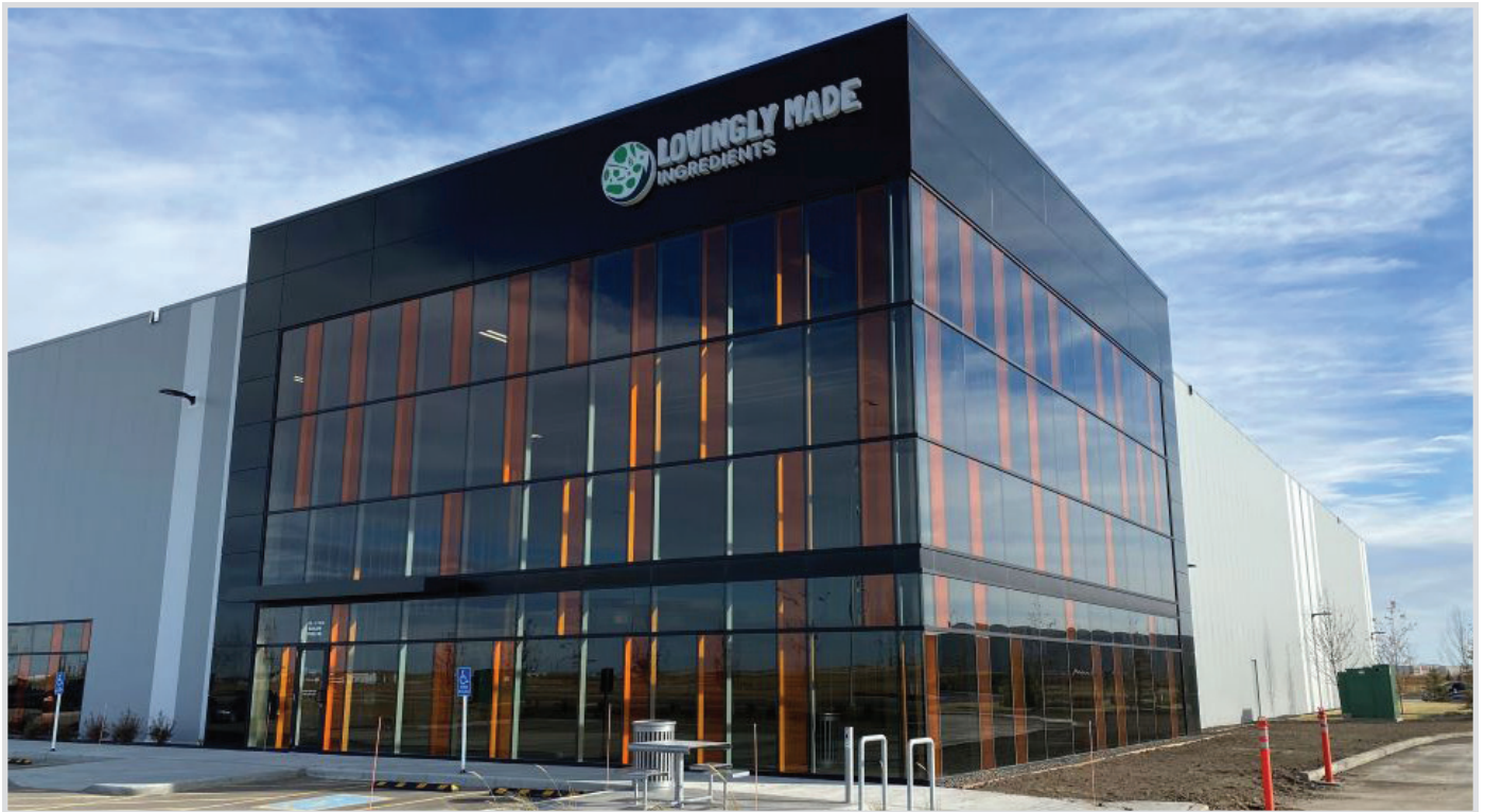
The Lovingly Made Ingredients facility in Calgary started production in March.
